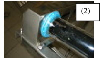
(1) Introduce carefully the tube into the hole of the tank and turn slowly in the watch direction, until the tube gets inside, approx 5 cms and introduce it turning into watch opposite direction until it gets strongly fixed into its base (2).
